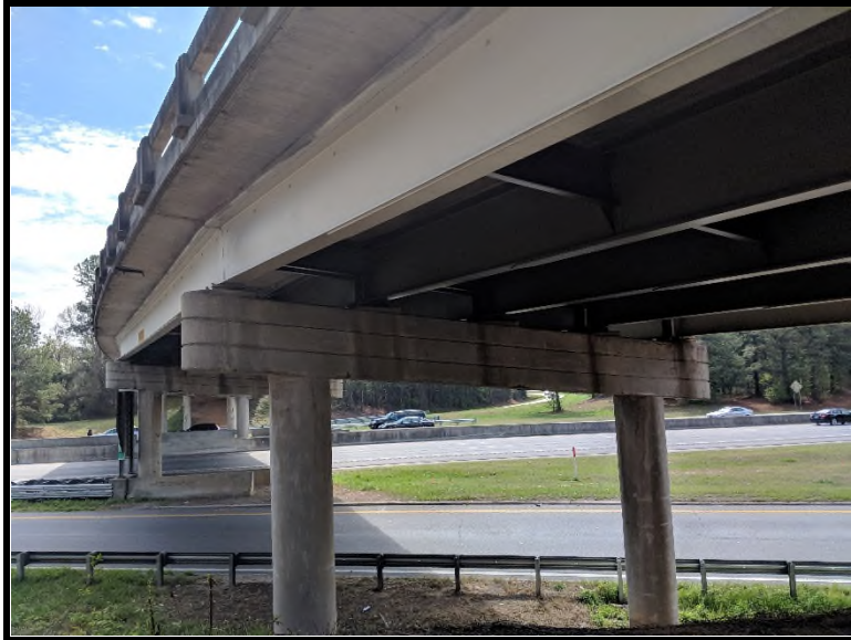
3 View of the underside of the bridge. Shows concrete decking, steel beams, and concrete piers.
