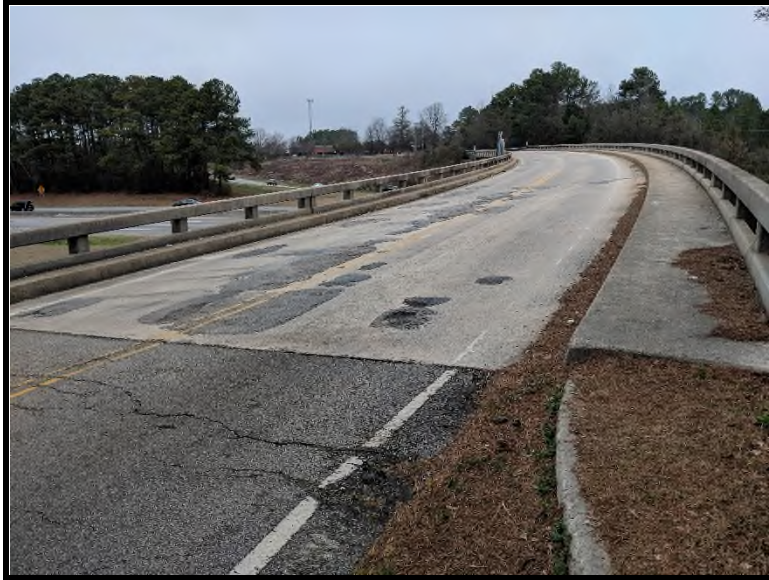
1 View of the Browning Road bridge over I-20.
