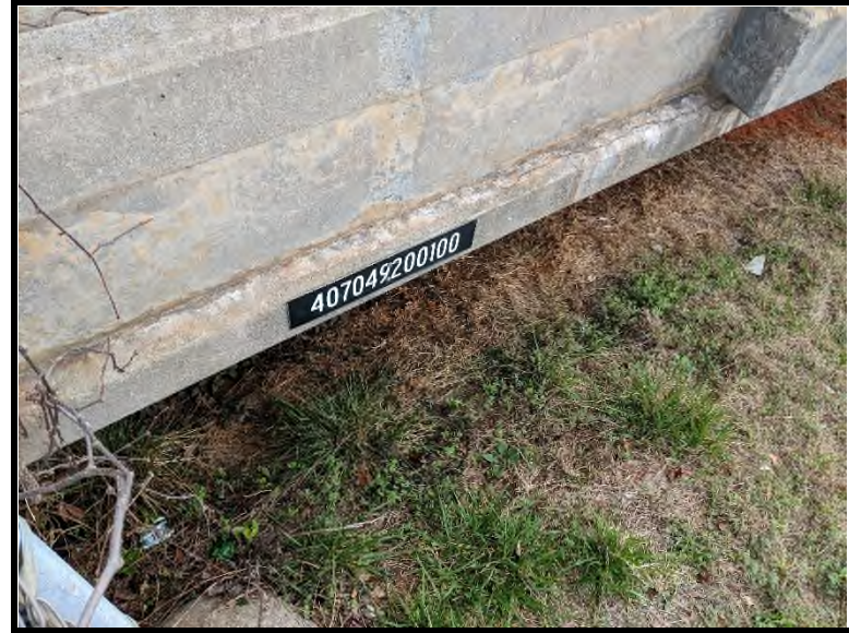
2 The bridge is identified as structure # 407049200100.
